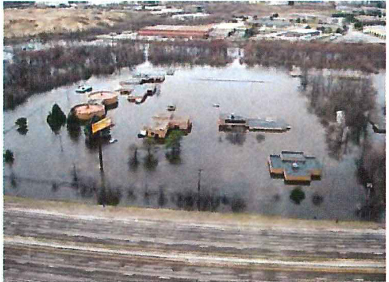
The flooding of the Warwick WWTF on March 30, 2010, resulted in $15 million in damages
